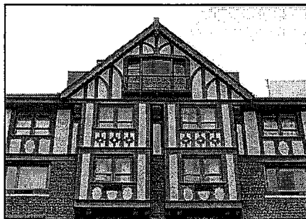
Alex Johnson Hotel, window detail, east elevation
